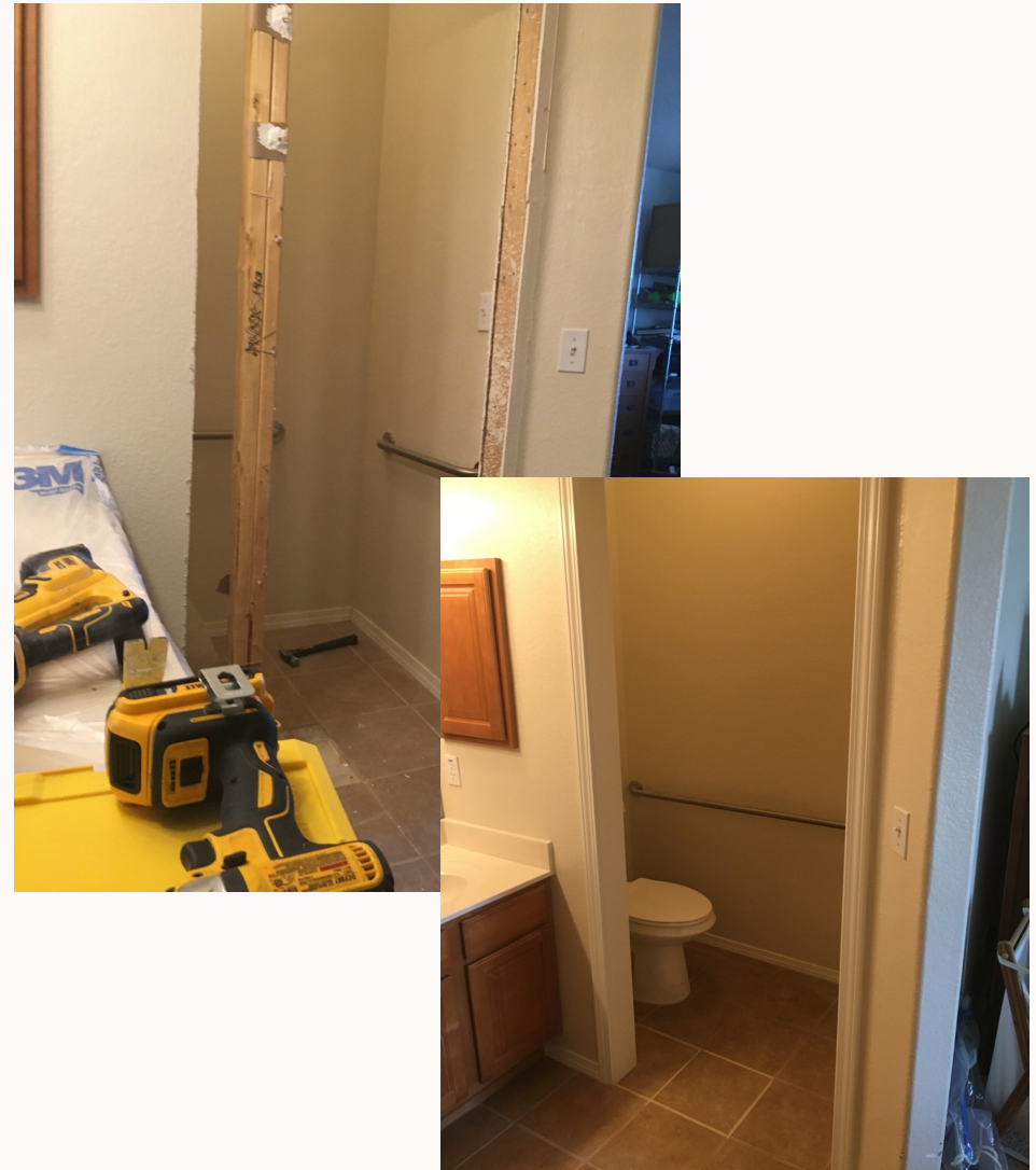
Photos of a door widening project completed by the HEART Carpenter, Steve Selgado.
